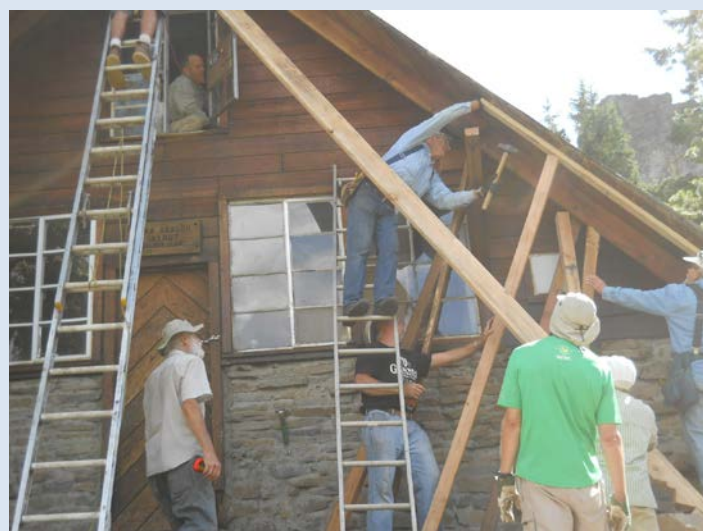
Repair Team wrestles with north side barge rafter and supports.
