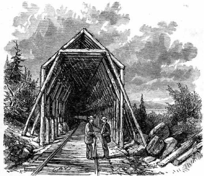
Section of Snow-shed.
