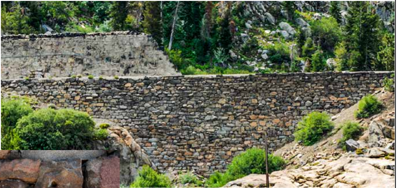
Above: China Wall, constructed by Chinese railroad workers. The stones fit perfectly with no mortar.
