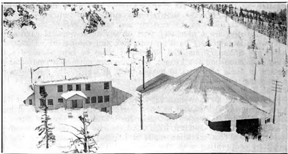
BUNKHOUSE AND TRUCK SHED AT DONNER SUMMIT, NEVADA COUNTY
