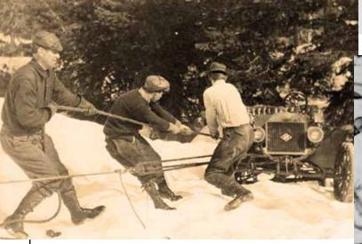
Note the 150' of 1" rope wrapped around the tires to give the car better traction.
