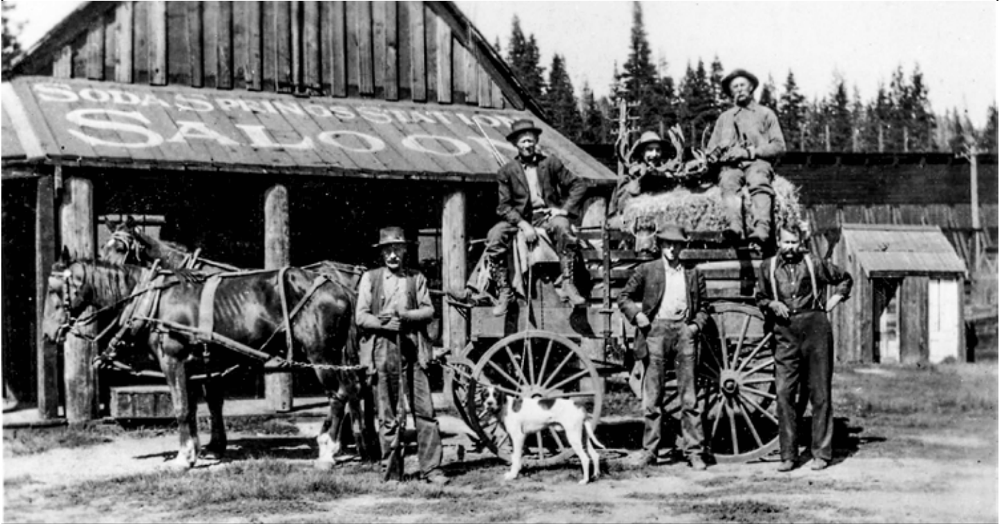
Soda Springs Station Saloon about 192. Note the snowsheds in the back.
