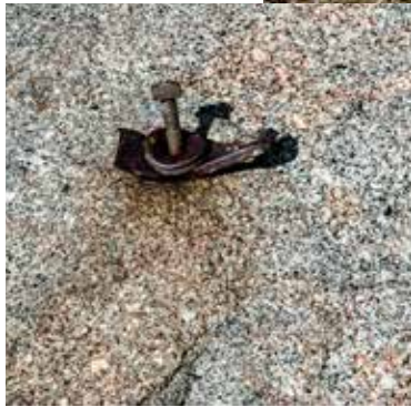
Bolt in the granite to which steel cable was attached to prevent the station from blowing away.
