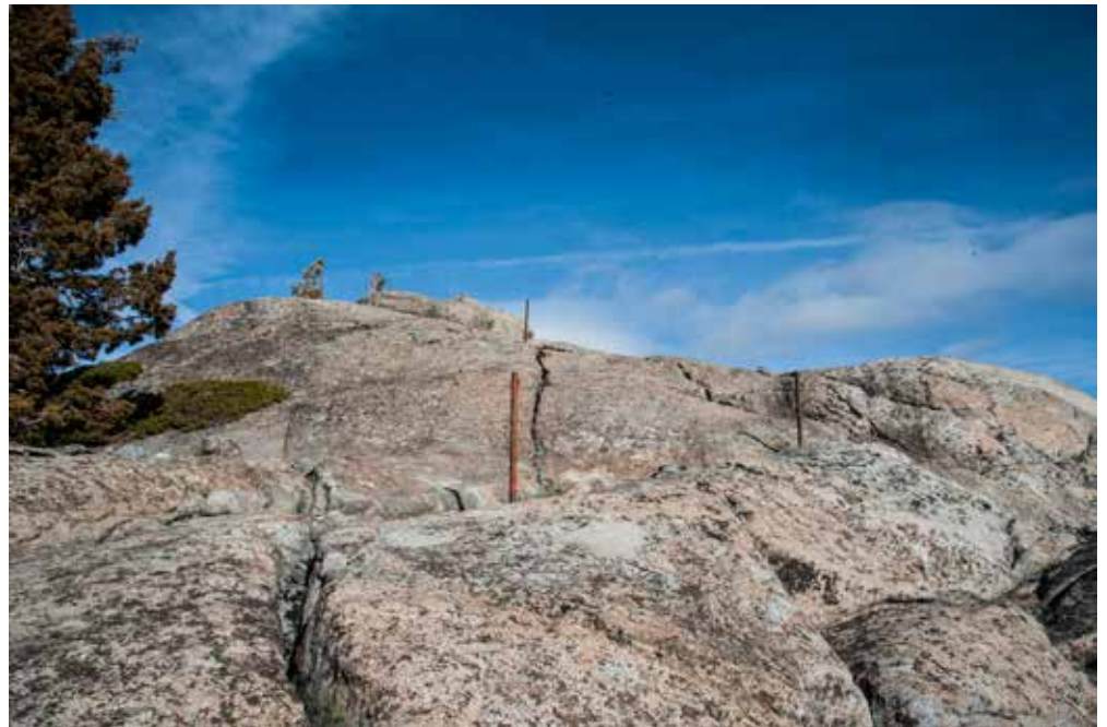
Bolt in the granite to which steel cable was attached to prevent the station from blowing away.
